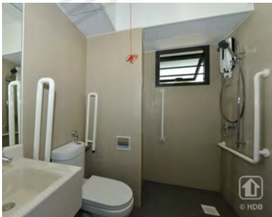
Wheelchair accessible bathrooms fitted with grab bars.
