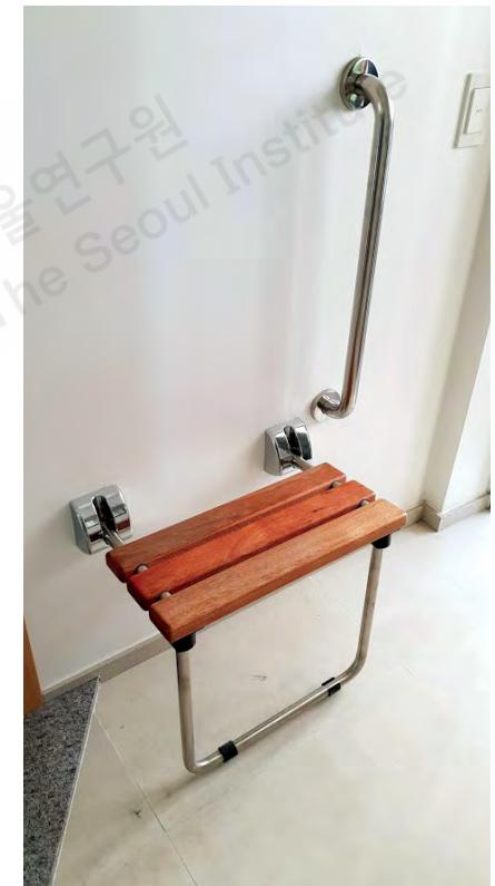
Folding patio chairs with handles for residents to put on their shoes.
