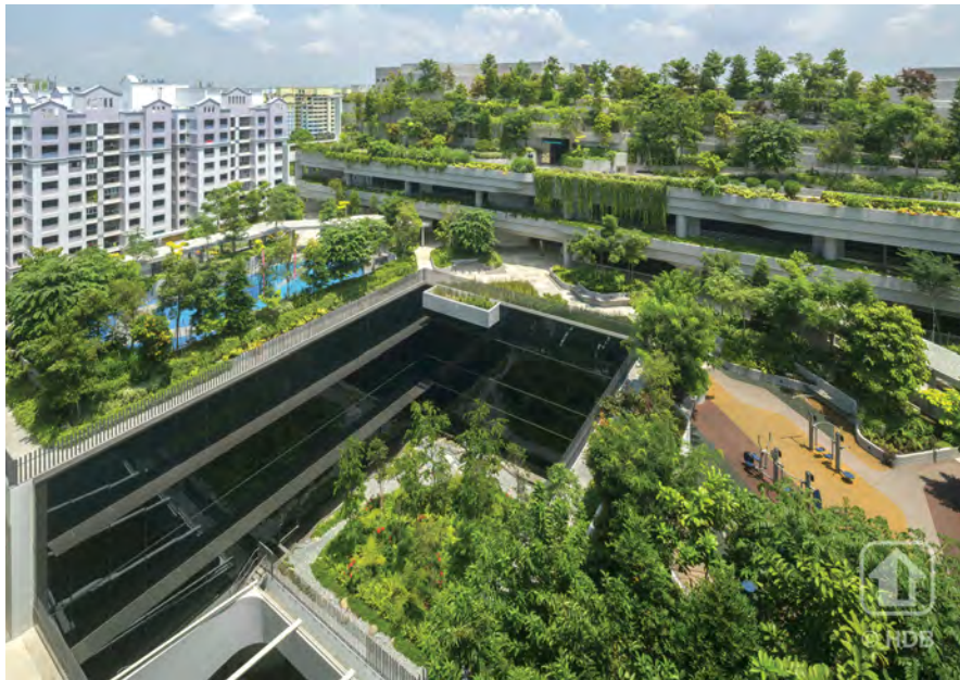
The tiered design of the community farm and gardens enables more greenery to be incorporated into the building, offering residents a lush and green environment which evokes the “kampung” feel of yesteryear.
